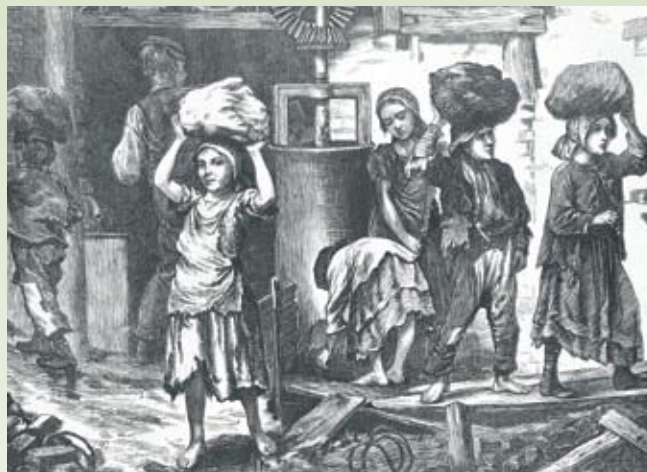
Figure 5-13 These children are carrying clay that will be used to make bricks. Child labour ended only when countries introduced compulsory education. Children who, by law, must be in school cannot also be at work.
