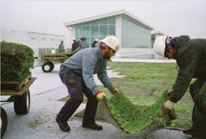
Figure 12-21 William McDonough designed the huge roof of the Ford Rouge Center truck factory in Dearborn, Michigan. It has been planted with a drought-resistant groundcover called sedum. The sedum grows in a four-layer mat of vegetation that collects and filters stormwater runoff (right). The roof helps cool the atmosphere in the surrounding community, absorbs carbon dioxide, and creates oxygen.
